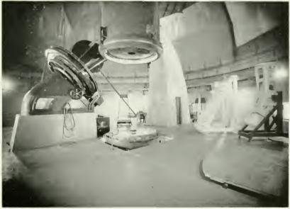
The hoist for removing the mirror for silvering
